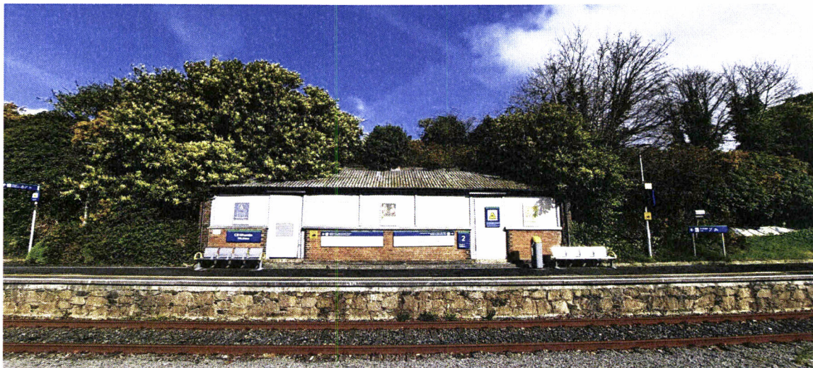
Platform 2 waiting shelter, view across running lines from Platform 1
