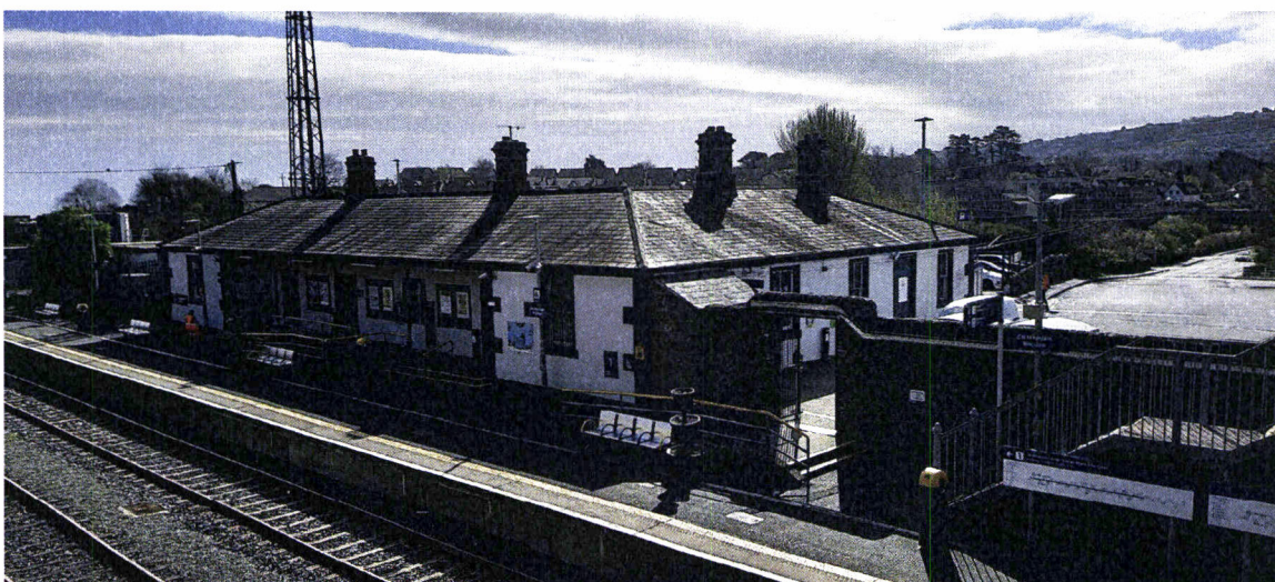
Elevated closer view of Platform 1 main station building from footbridge, boundary wall and gated entrance View looking south east 2026-04-01.
