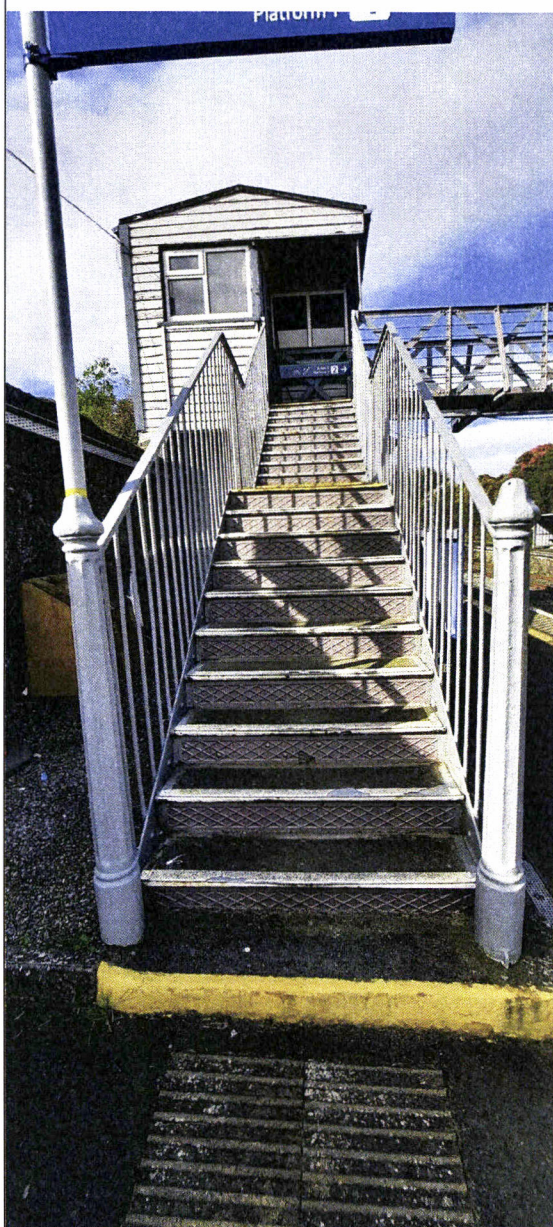
Footbridge access staircase from Platform 1, signal cabin at head of stairs
