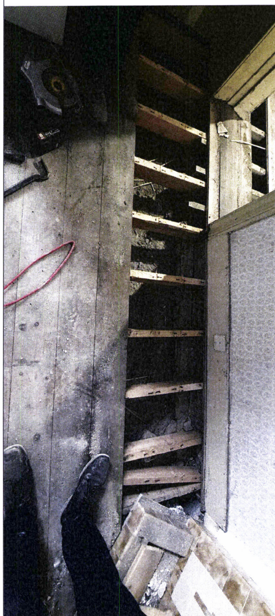
Interior, exposed former stair/floor void showing timber joists and construction debris
