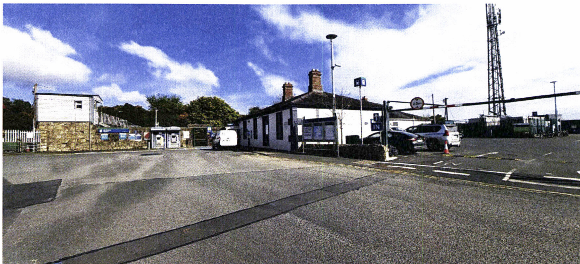
Station forecourt, entrance approach (alternative angle), height-restriction barrier and telecommunications mast
