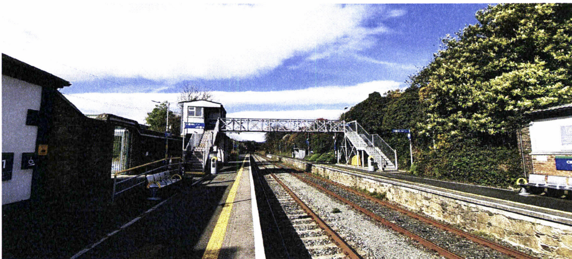
Platform 1, looking towards footbridge and signal cabin
