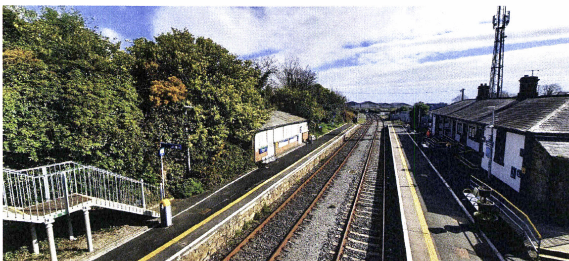
Elevated view from footbridge looking down on Platform 2 waiting shelter and Platform 1 building
