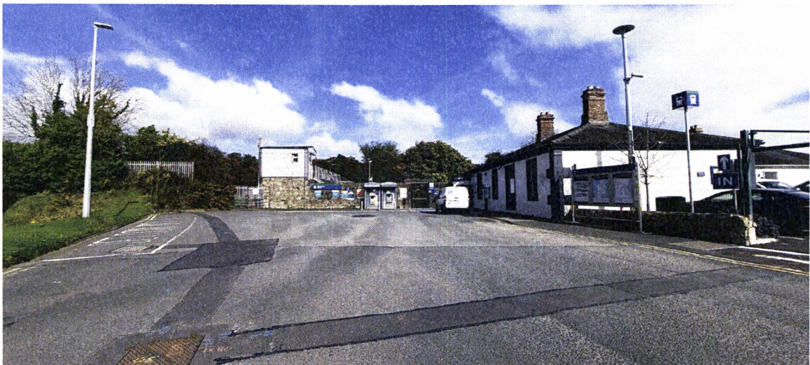
Station forecourt, entrance approach with ticket vending machines View Looking North to down platform entrance. 2026-04-01.
