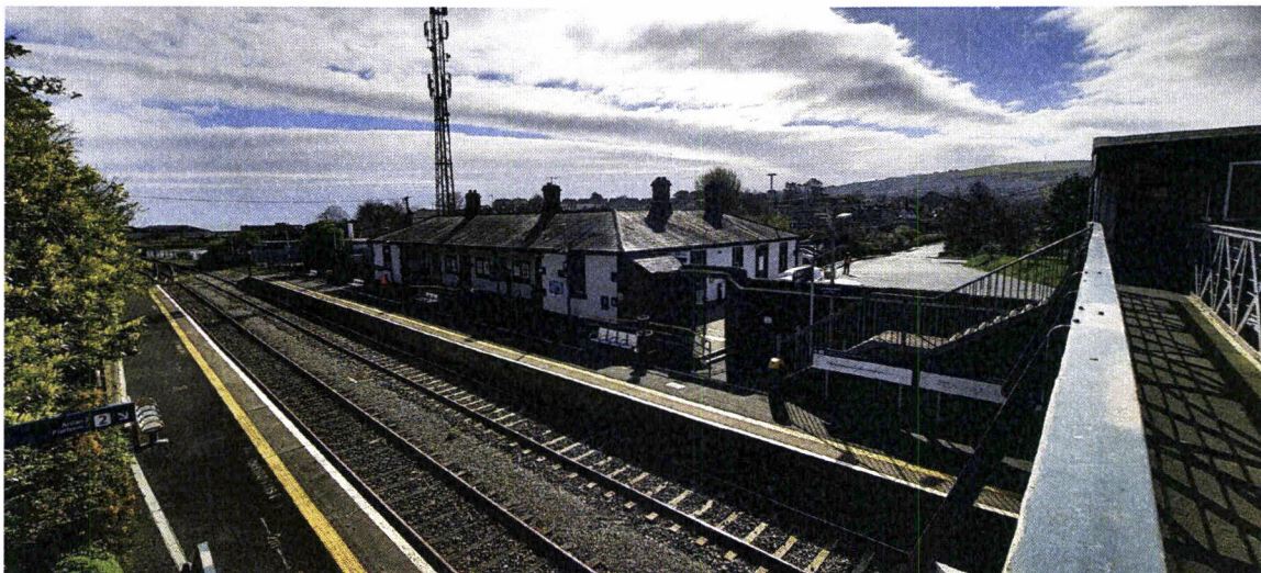
Elevated view from footbridge looking down on Platform 1 main station building, hills beyond View looking south east 2026-04-01.
