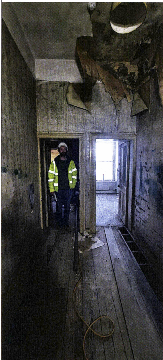
Interior corridor (alternative angle), hanging wallpaper, door architraves, exposed floorboards, site engineer in in background for scale 2026-04-01.
