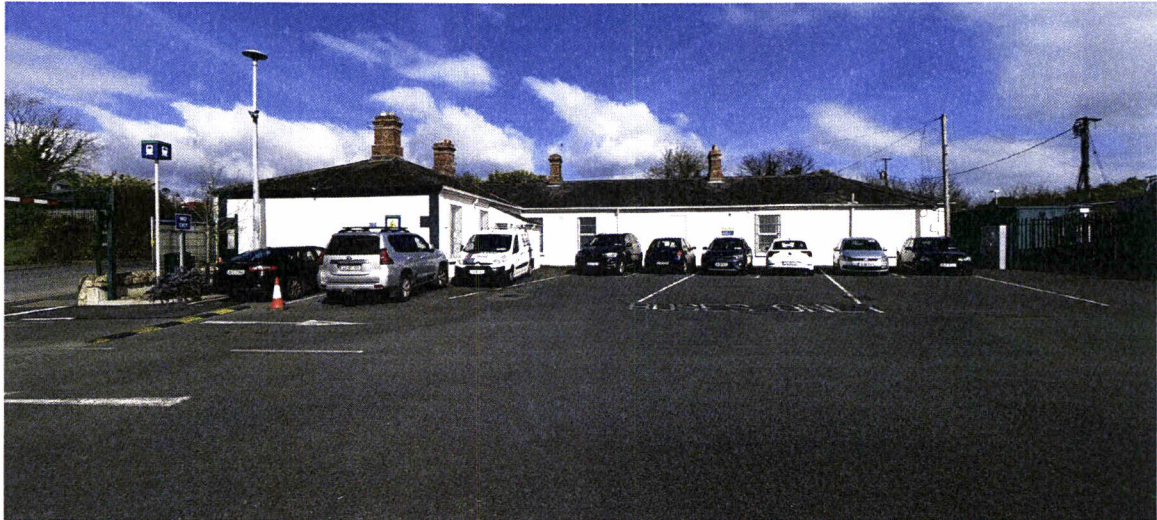
Station forecourt and car park, rear elevation of main station building View Looking north to rear (south elevation)]. 2026-04-01.
