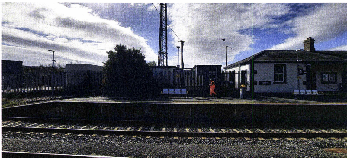
Platform 1, ground-level view towards footbridge and signal cabin
