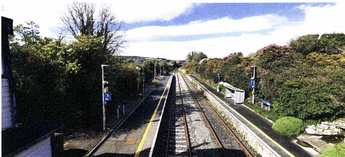
Elevated view from footbridge looking along Platforms 1 and 2
