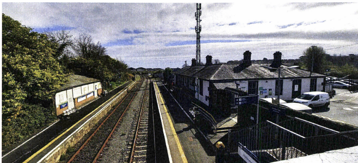
Elevated view from footbridge looking down on Platform 1, main station building and car park View looking east or in 'up' / Dublin direction 2026-04-01.
