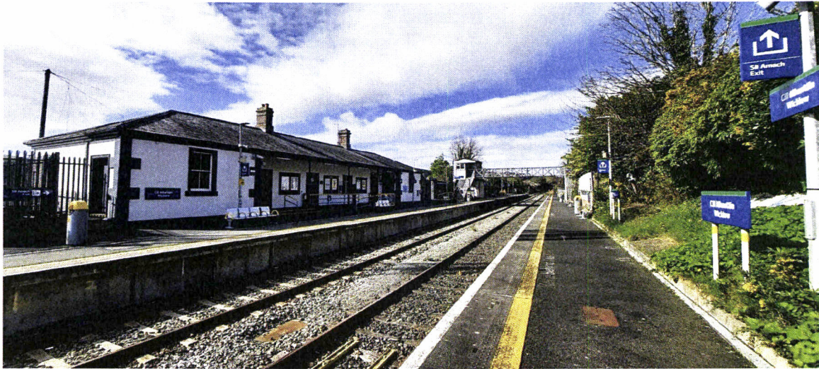
Platform 1, ground-level view along main station building towards footbridge
